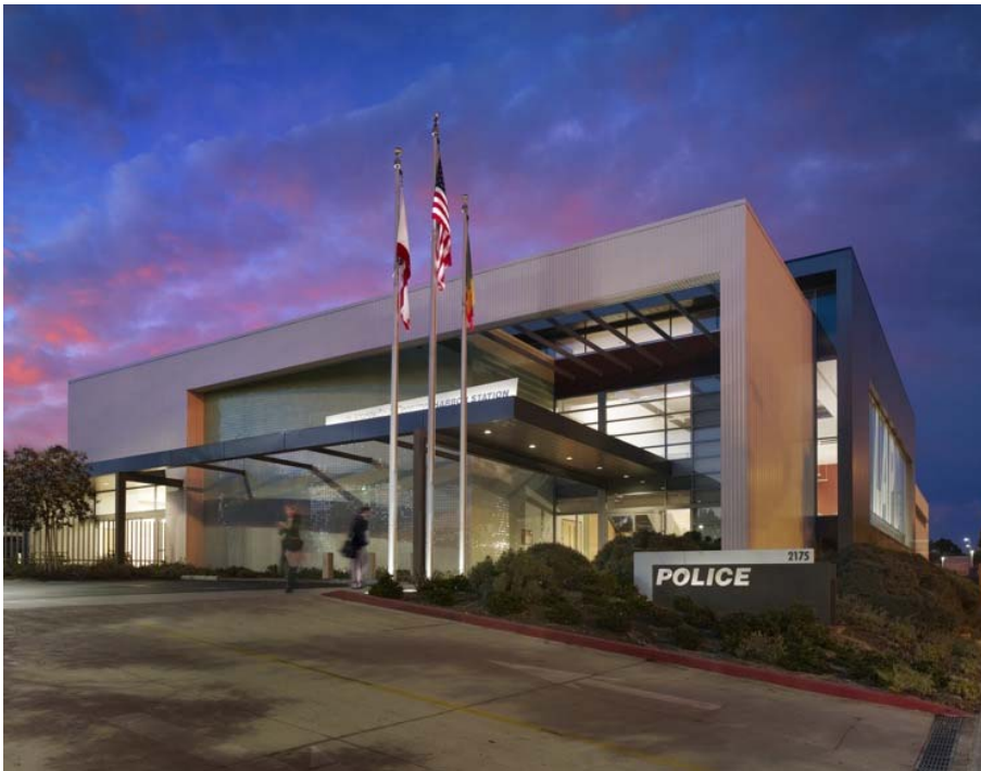
LAPD Harbor Replacement Station and Jail Perkins + Will, Pinner Construction Co., Inc., City of Los Angeles, Bureau of Engineering Prop Q Program
