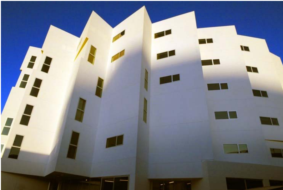
The New Carver Apartments Michael Maltzan Architecture, Inc., Westport Construction Inc., Skid Row Housing Trust
