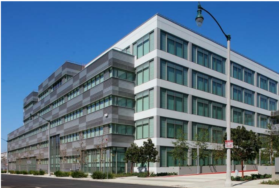
Horizon at Playa Vista Johnson Fain, Morley Builders, Lincoln Property Company
